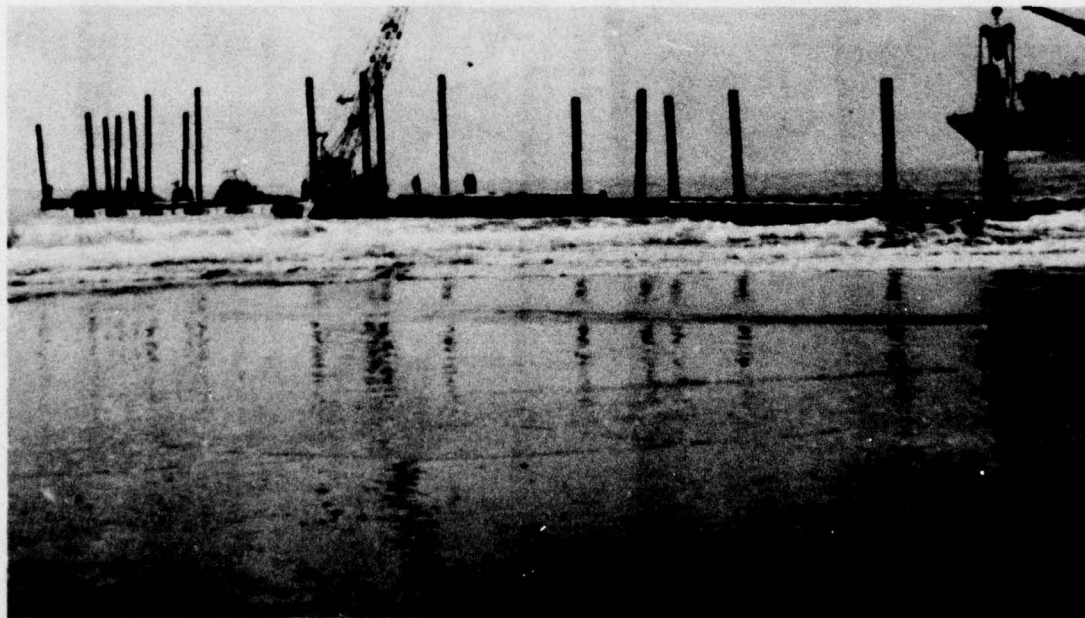
Figure 11. Transferring chain jacks with hydraulic crane during pier construction.
