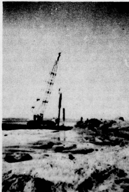
Figure B-3. Driving pile with DE-30 diesel pile hammer.
