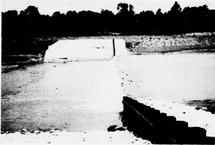
Figure 2. Item 30A weir
