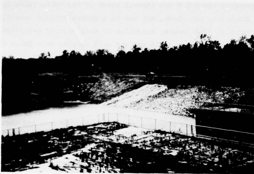
Figure 4. Little Sunflower Drainage Structure
