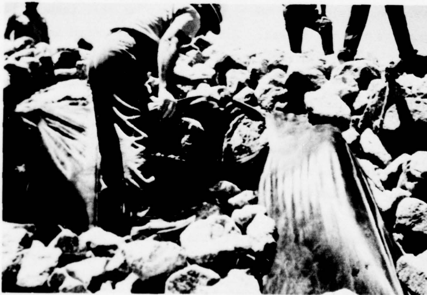
Figure 18. Erosion beneath cloth possibly prior to soil displacement Reach 1 - Weir 2
