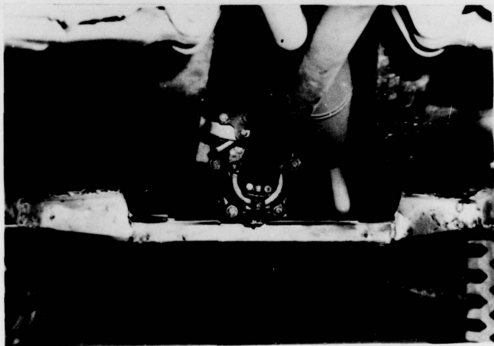
Photograph 6.4 - Capping of Cross Member Under Transmission as Per TM-9-2320-218-34.
