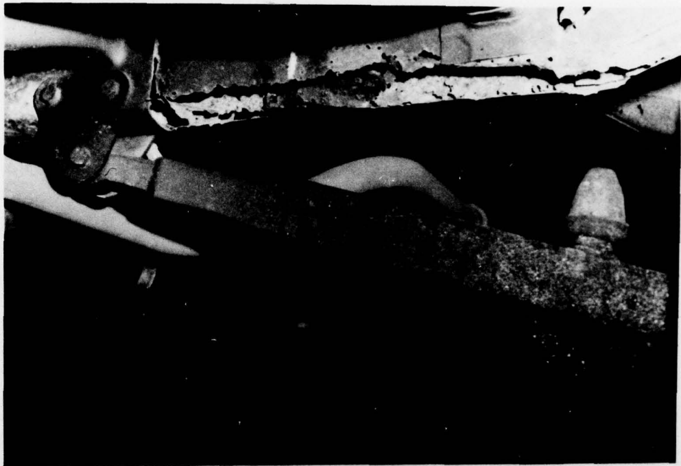
Photograph 6.1 - Typical Example of Severely Rusted Rear Cross Member.
