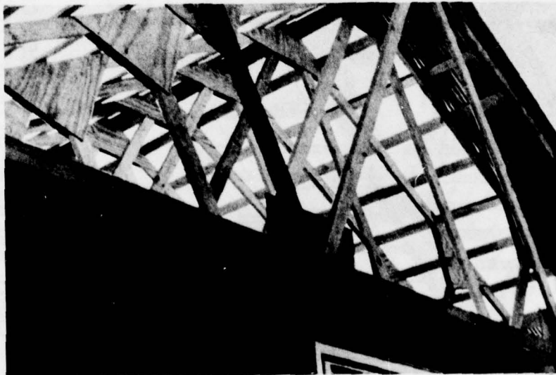
Figure 14. Nailer strips on roof trusses.
