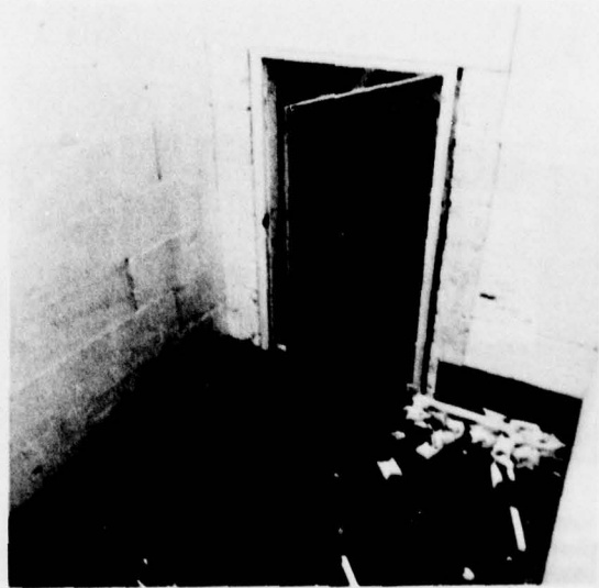
Figure 8. Door unit in utility room.
