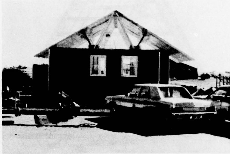
Figure 13. Wood truss roof support system.
