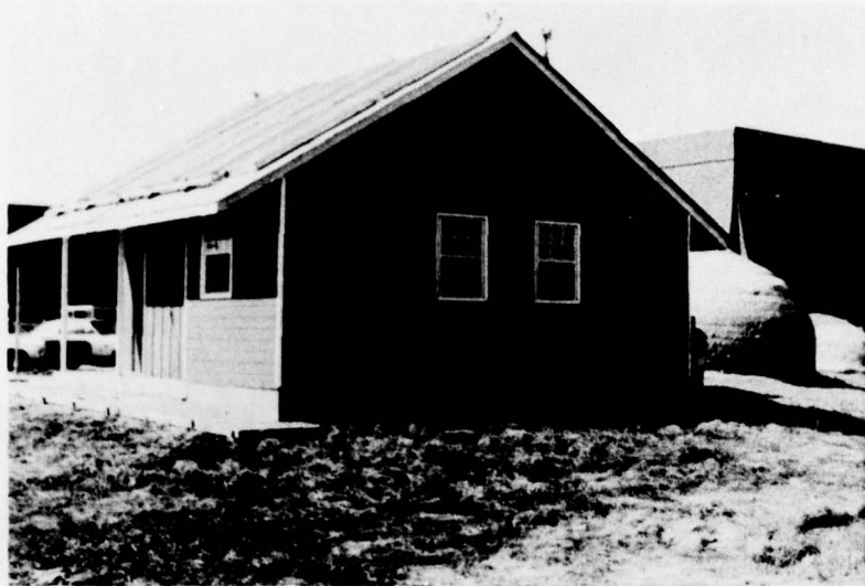
Figure 15. Completed structure with collector panels on south-facing roof.
