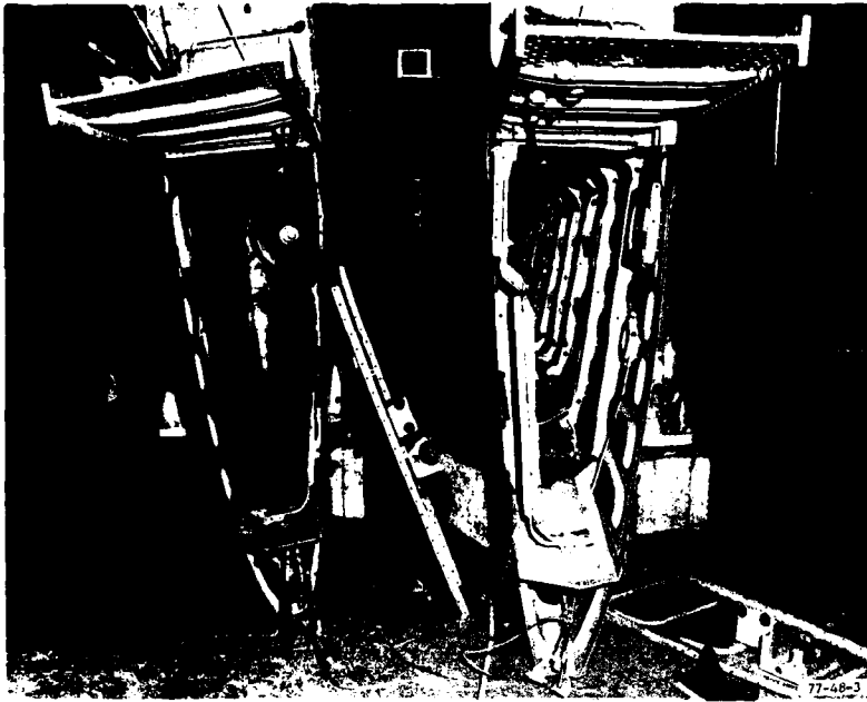
FIGURE 3. INSTALLATION OF TWO-PLY FUEL TANK
