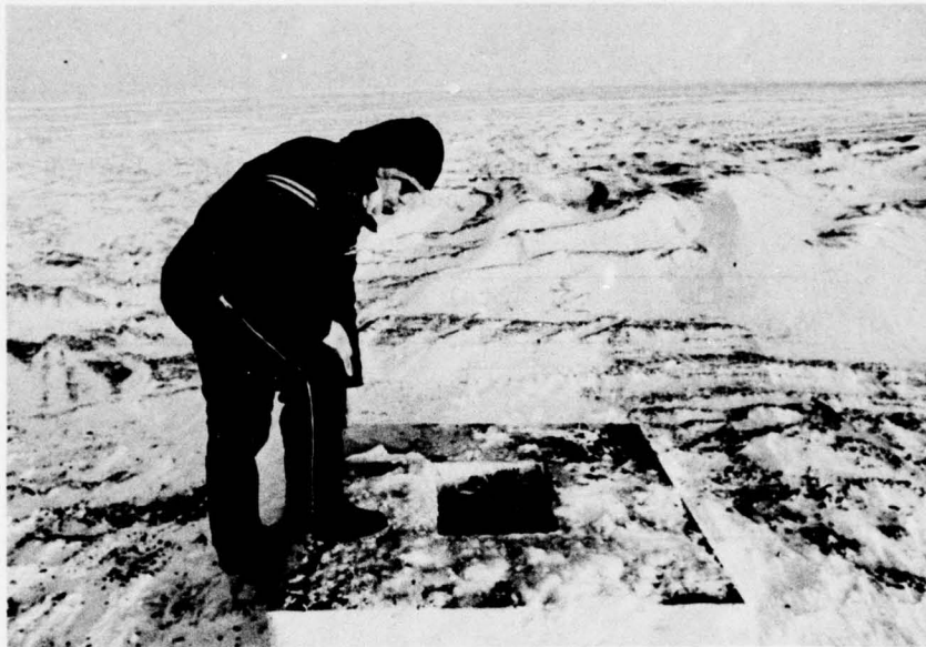
Figure 3. Surface water well in the gravel of the spit. Note well is enclosed to protect well from contamination.
