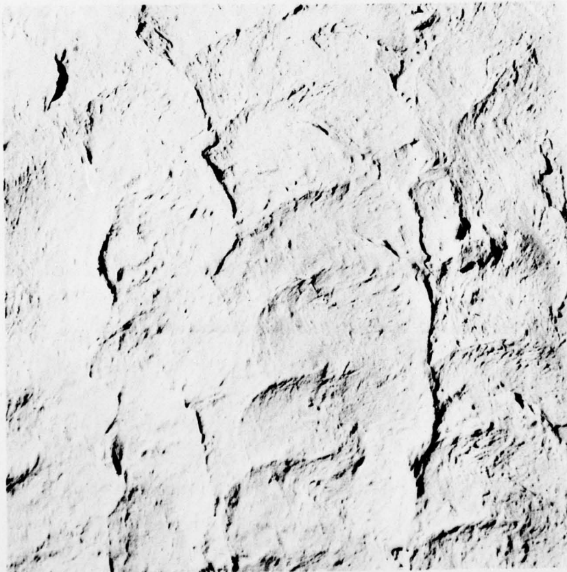
Figure 8-31. A stucco effect can be obtained with a standard paring trowel.
