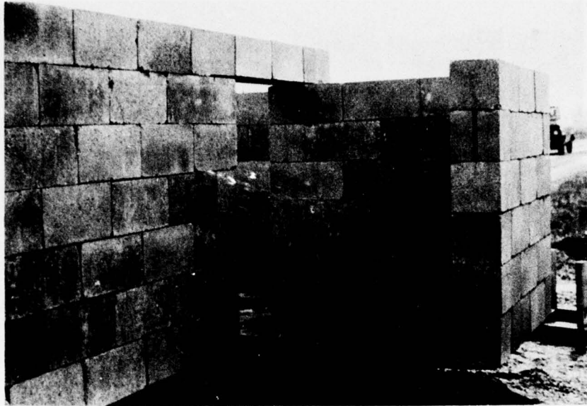
Figure 2. Blocks can be laid to a height of 10 ft (3 m) before applying the glass fiber cement parging.
