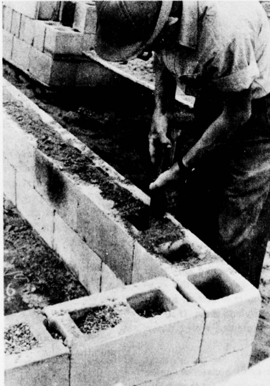
Figure 4. Protection from small arms fire can be achieved by filling the cells of the blocks with soil, gravel, mortar, or concrete.
