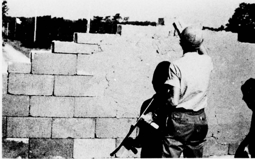
Figure 3. Stacked block being parged with glass-fiber-reinforced cement.
