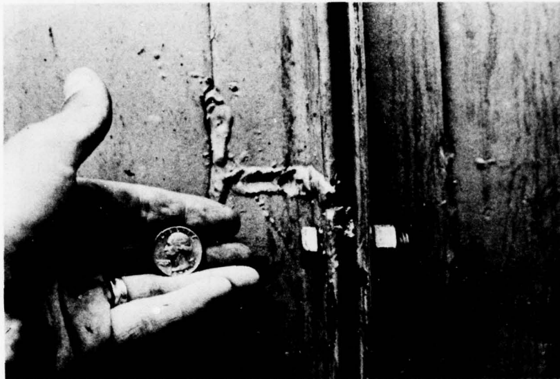
Figure 8. Bolted assembly of furnace sections 1 and 2.
