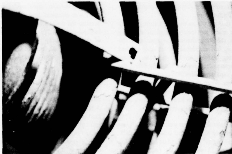
Figure 26. Spalling of heat exchanger surface.
