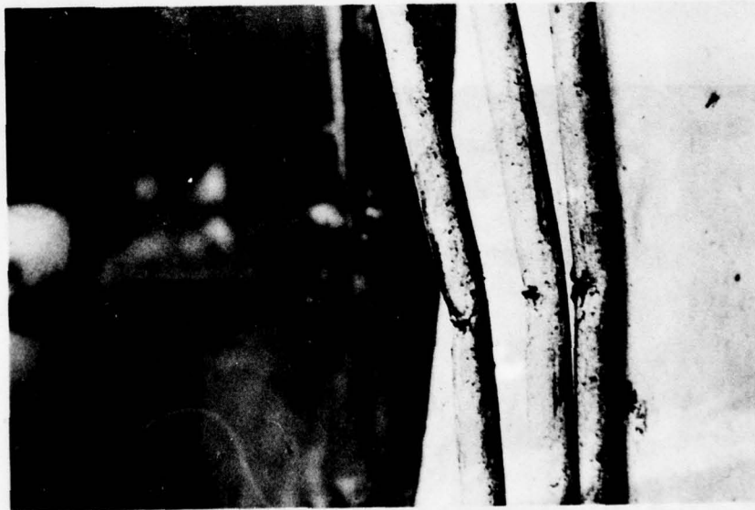
Figure 22. Impingement of rear inspection door on hydraulic lines.
