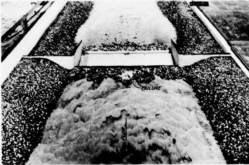
a. Looking downstream
