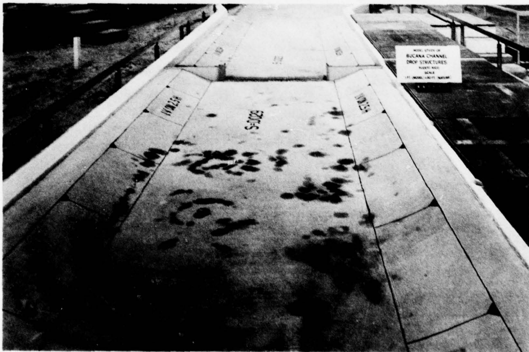
b. Drop structures
