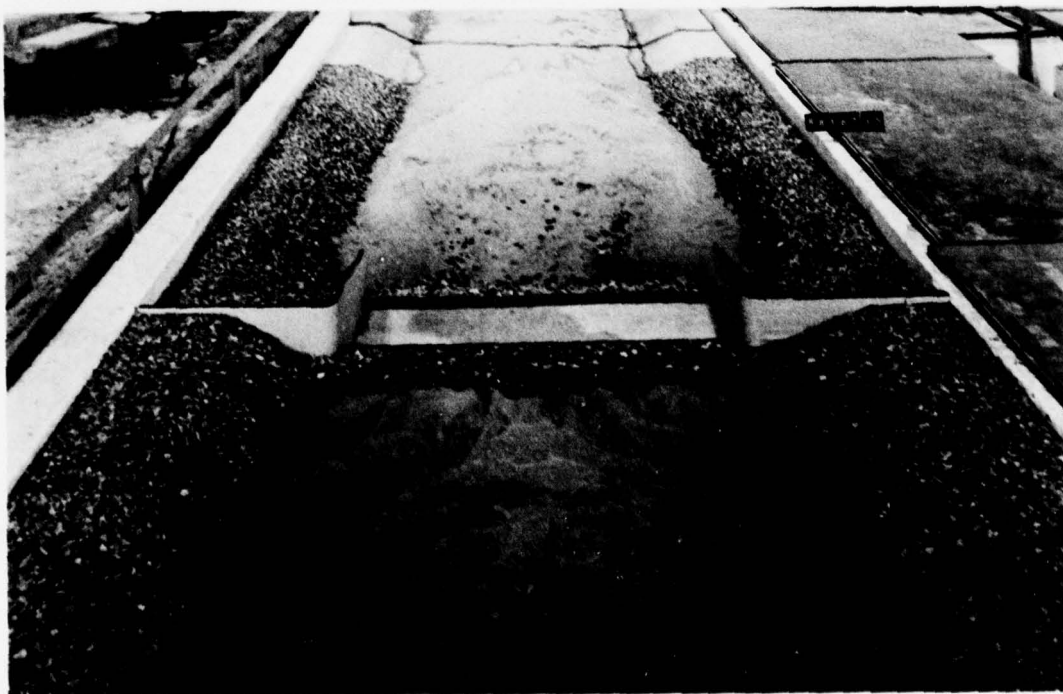
Photo 10. Drop structure 4 (design 4); type 8 riprap plan (recommended) after 1-hr (prototype) operation with 24,700-cfs flow
