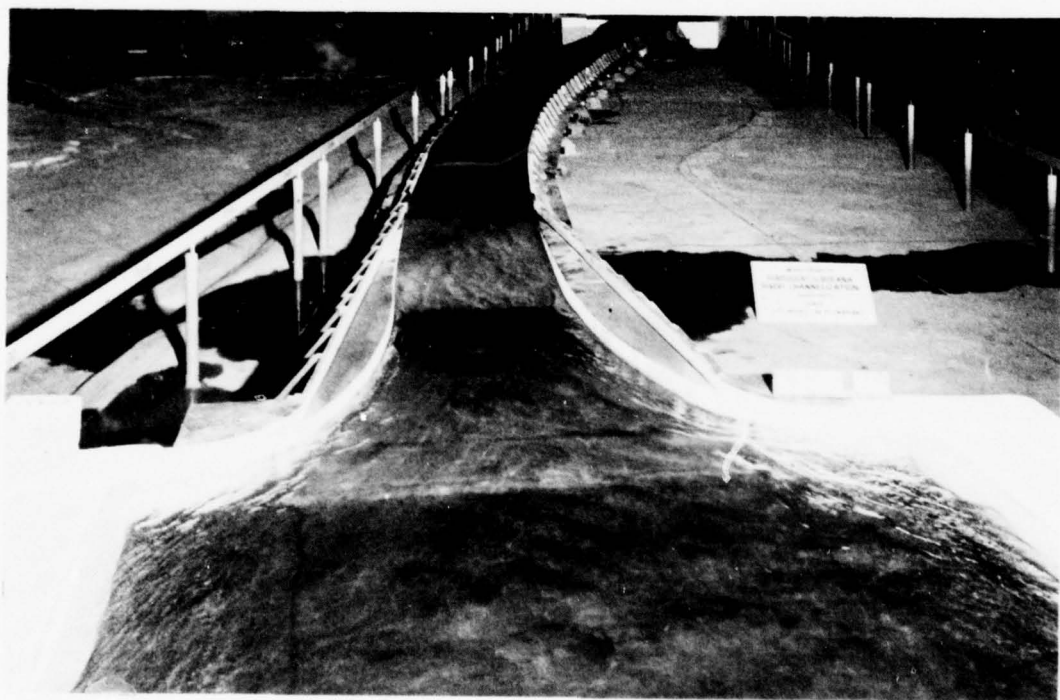
Photo 14. Bucana Channel design 3 transition at sta 157+81; design flow 28,900 cfs, bottom slope 0.0514
