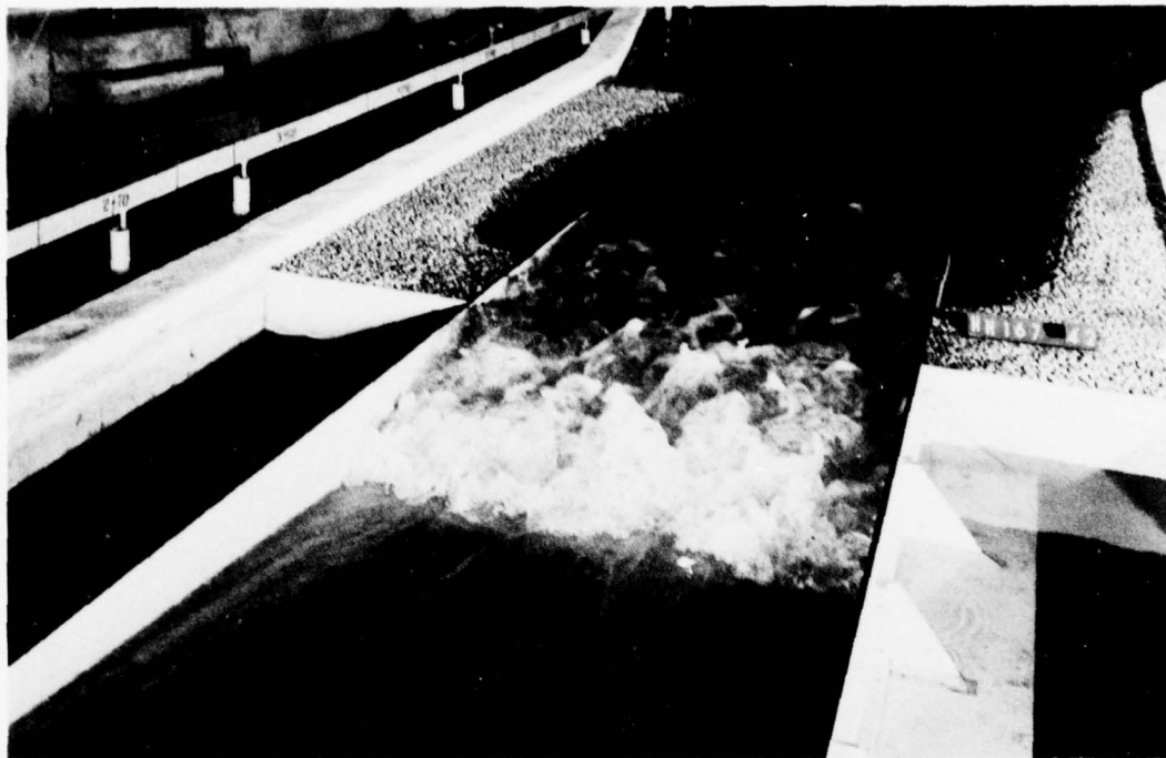
Photo 17. Stilling basin B-2 (original design); design flow 28,400 cfs, tailwater el 56.3
