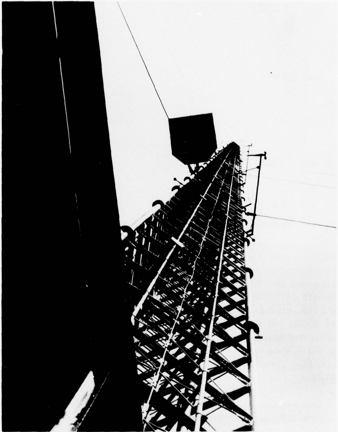
Figure 1-2 View up southwest face of NSSL-KTVY meteorological tower. Conduit bridge is in left foreground.
