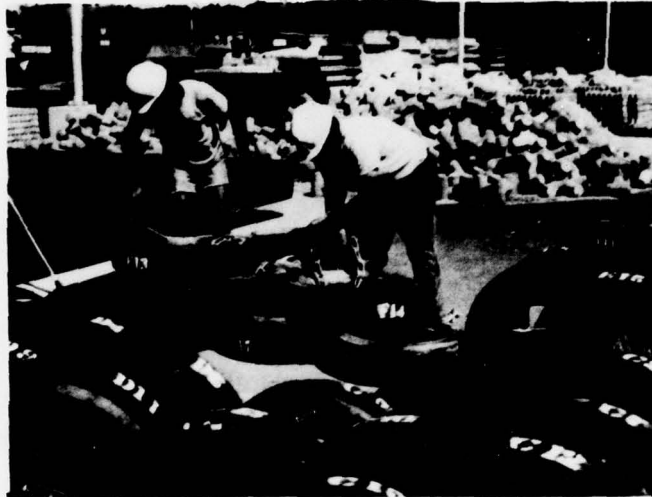
a. Threading the chain through the tires as they are stacked.
