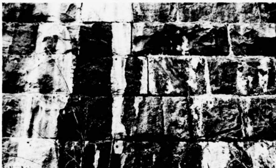
CRACK AND SEEPAGE AT NORTH END OF DAM
