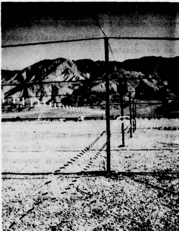
Figure 3 View of E arm column looking North. Note DC control line cables on ground at base of pole.
