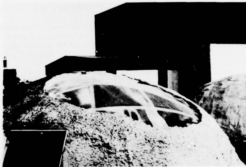
Figure 2. Aluminum screen wire in place.
