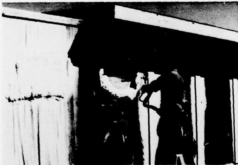
Figure 12. Application of foam to the edge of the hole first.
