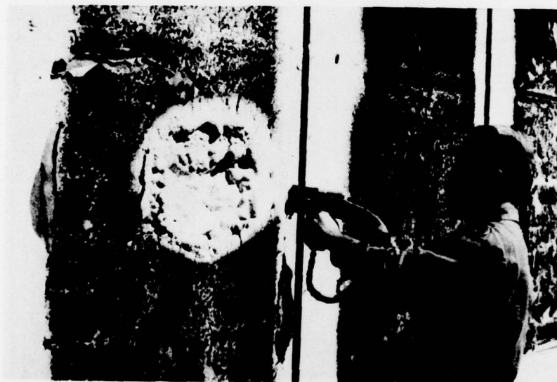
Figure 14. Completing the patch.
