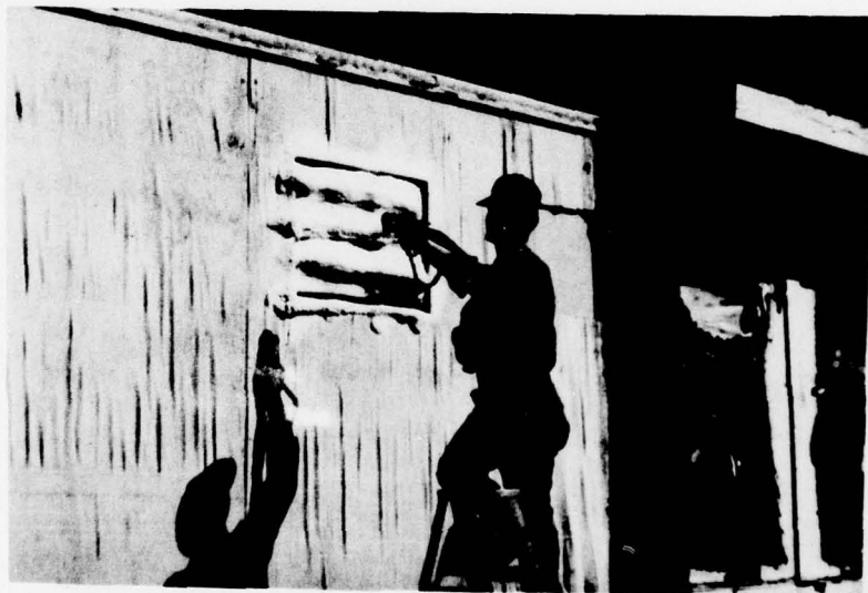
Figure 10. Spray foam being applied to insect screen substrate to make patch.
