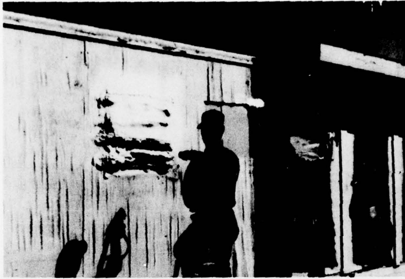
Figure 11. An excess of foam may be applied and trimmed off, if desired.
