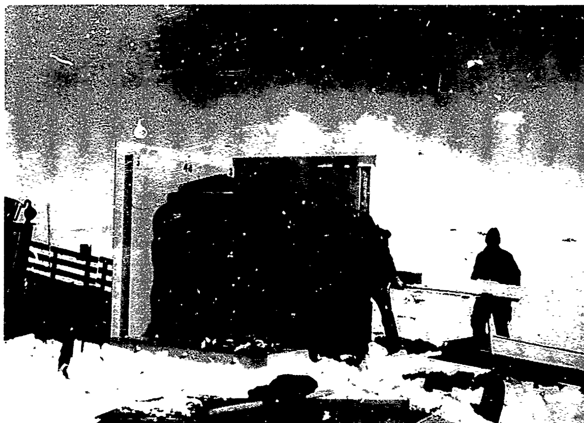
Figure 2-6. Erecting Prefabricated Building Around the RTG; Nodwell Vehicle is in Hole Dug to Facilitate Unloading of RTG.
