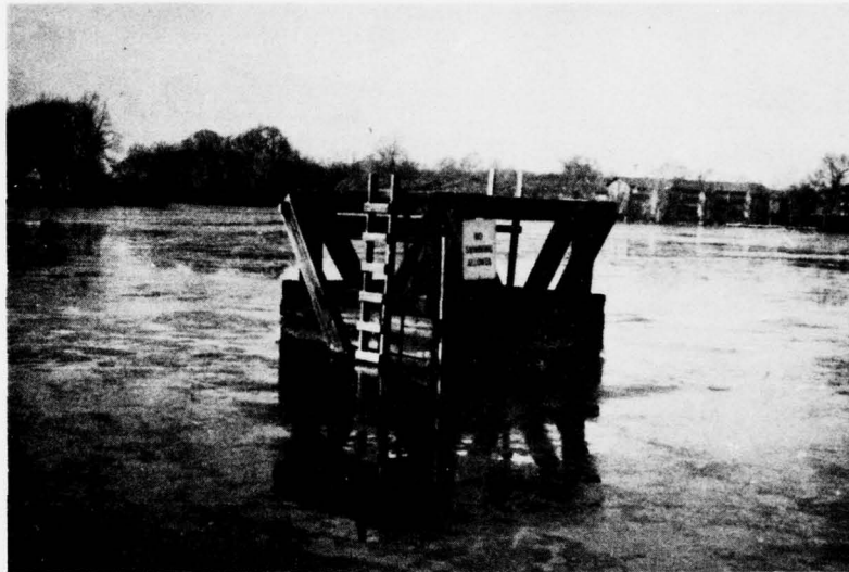
3. 13 Dec 77. View of sluice gate operating platform. Photo from left abutment area looking north toward upstream reservoir area.
