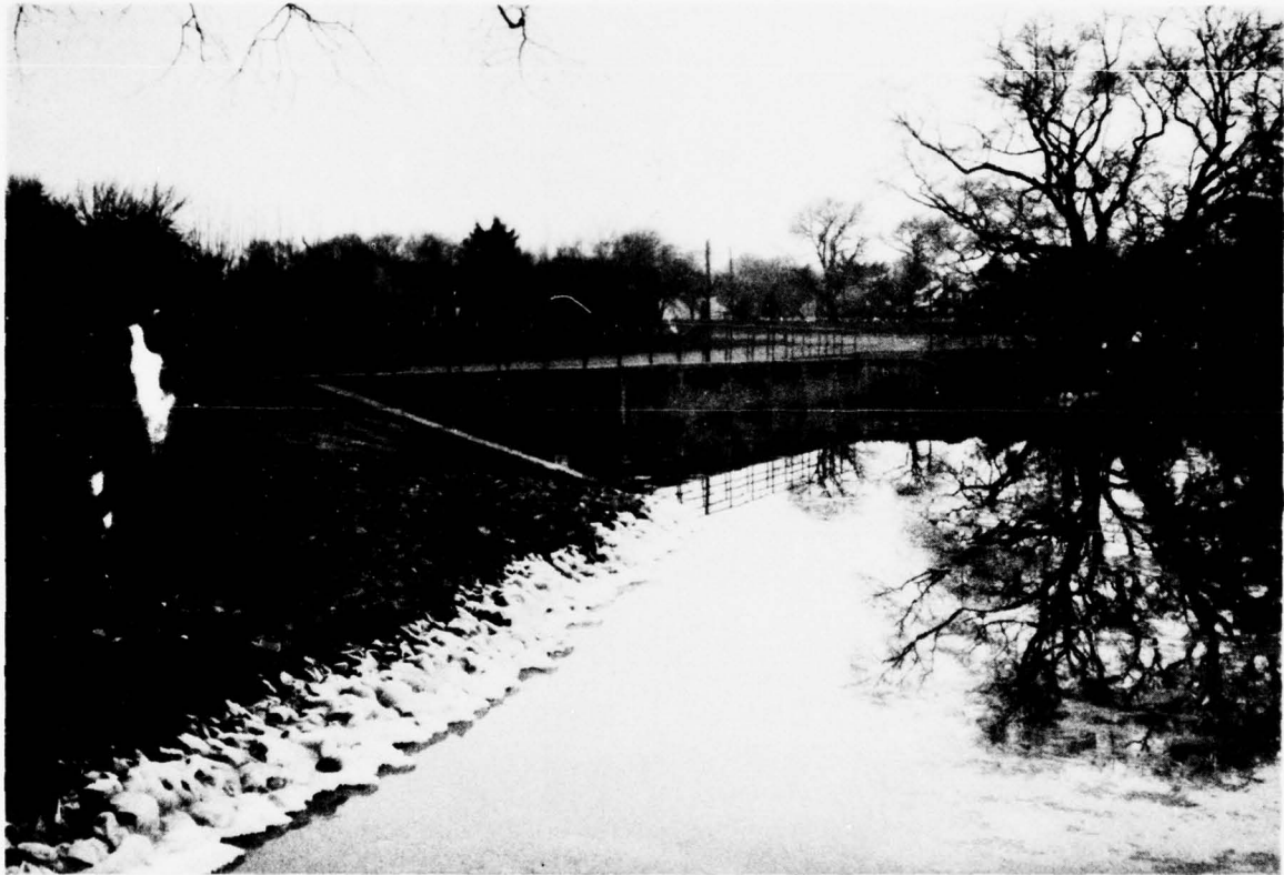
OVERVIEW PHOTO SILVER LAKE DAM VIEW LOOKING WEST FROM UPSTREAM OF LEFT ABUTMENT TOWARD RIGHT ABUTMENT
