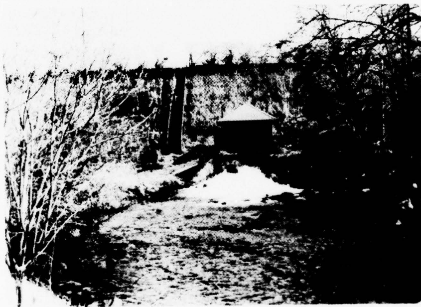
Photo 2 - Looking at dam embankment and low level outlet Gate House from downstream
