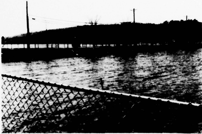
Photo 15 - View of upstream face of causeway dividing Woodcliff Lake into two parts; connected by a single barrel culvert 25-foot wide by 18'-9" high
