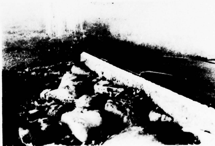
Photo 10 - Upstream face of spillway weir under spillway bridge showing approach stone protection, and abandoned and bent flashboard pins
