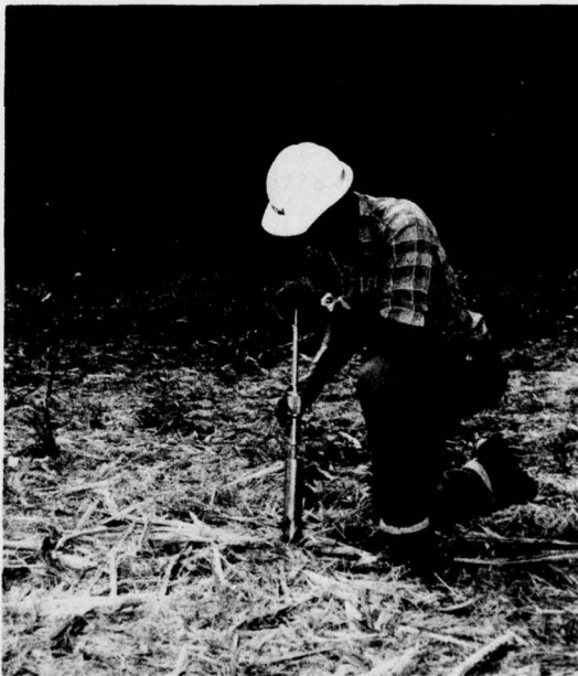
d. Applying hammer blows
