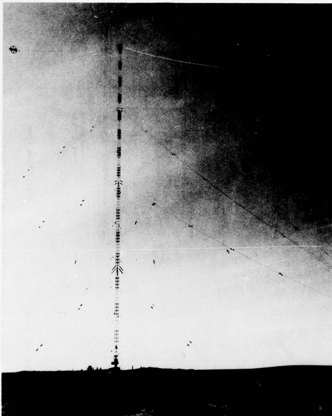
Figure 1. Guyed VLF antenna tower at the Hawes radio relay facility near Hinkley, Calif.
