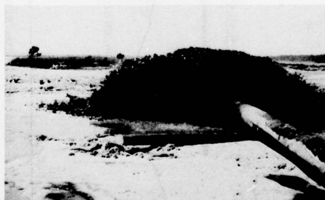
c. Pumping dredged material into the containment area
