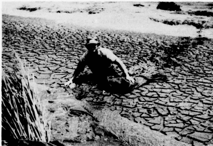
Figure 5. Sprigging smooth cordgrass ( Spartina alterniflora ) by hand in fine-grained unconsolidated dredged material
