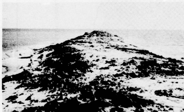
b. Close-up of dike, heavy clay material
