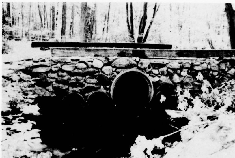
Photo 11 - Multiple culverts under private road downstream of dam.
