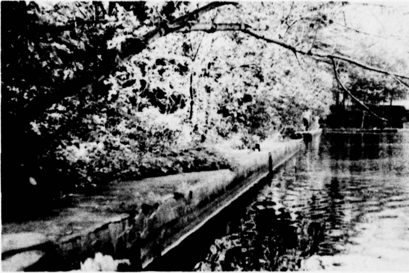
Photo 1 - View of dam, outlet notch and spillway from left abutment.
