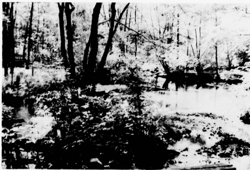
Photo 13 - View looking downstream from culverts.
