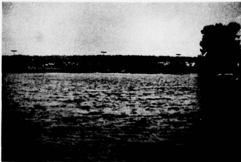
Photo 2 - View of dam and left abutment from upstream right shoreline.
