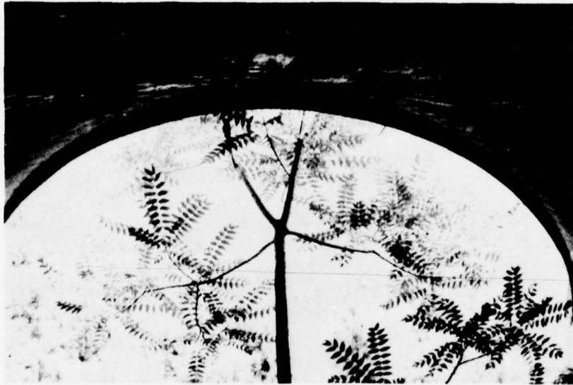
Photo 5 - Underside of top of arch.
