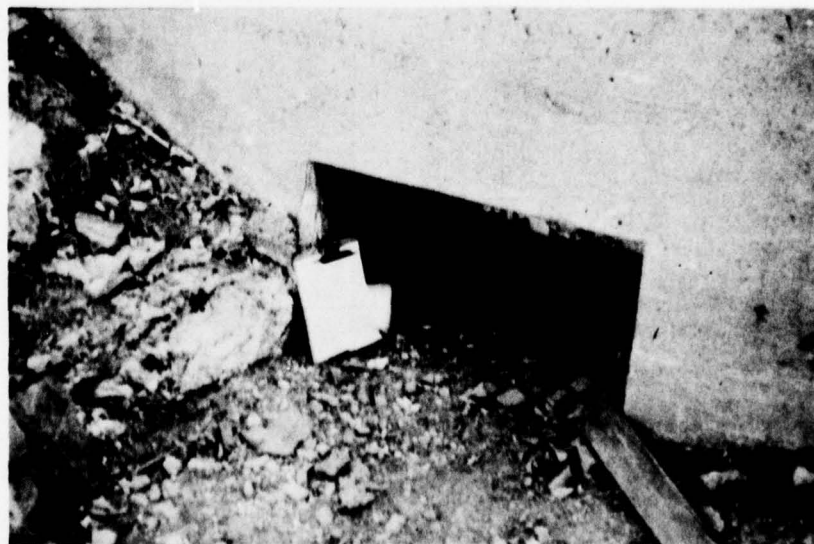
Photo 10 - View of spillway outlet opening.
