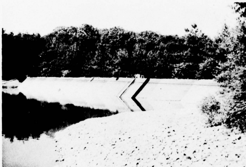
Photo 1 - Upstream view of dam from right shoreline.
