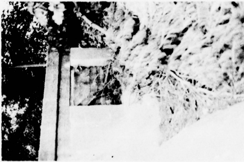
Photo 11 - View of spillway inlet box.
