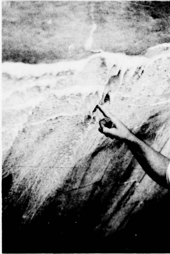
Photo 9 - Close-up view of leach deposits.
