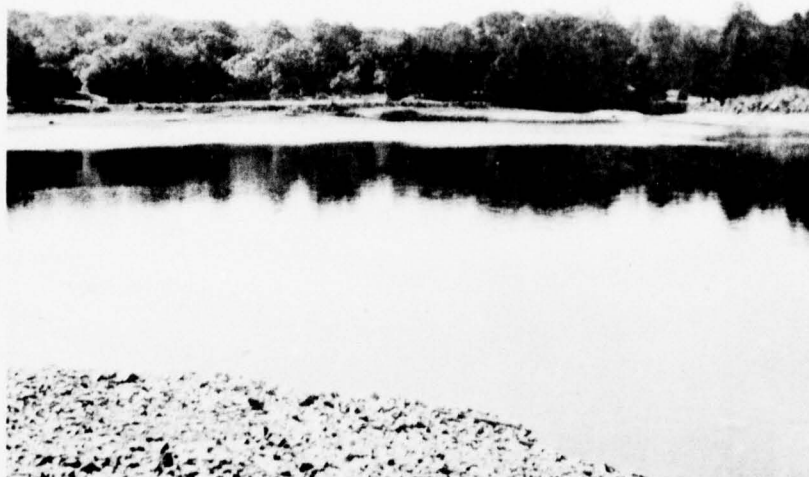
Photo 17 - New Street Reservoir and left shoreline.
