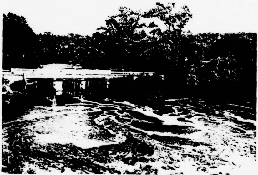
County Bridge downstream of Spillway July 1978
