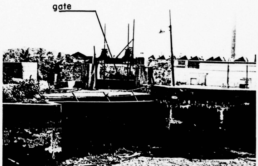
Inoperative gate to 9' Powerhouse penstock July 1978
