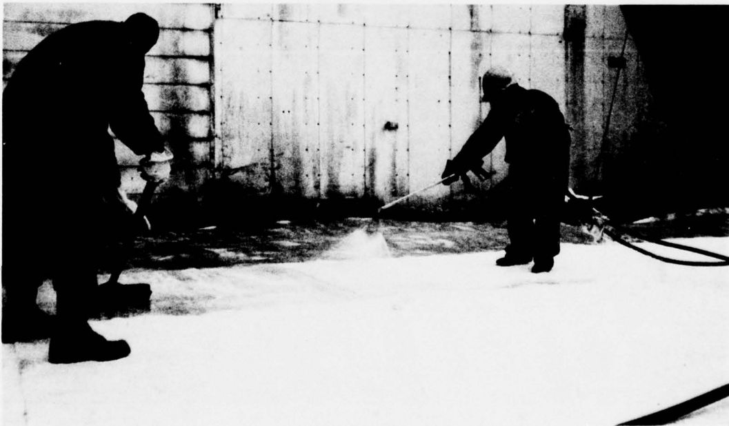
Figure 10. Resin spraying and fiberglass rolling operations.
