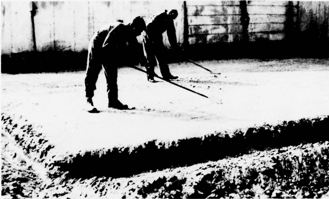
Figure 9. Removal of rocks and other objects in preparation for FRP construction.
