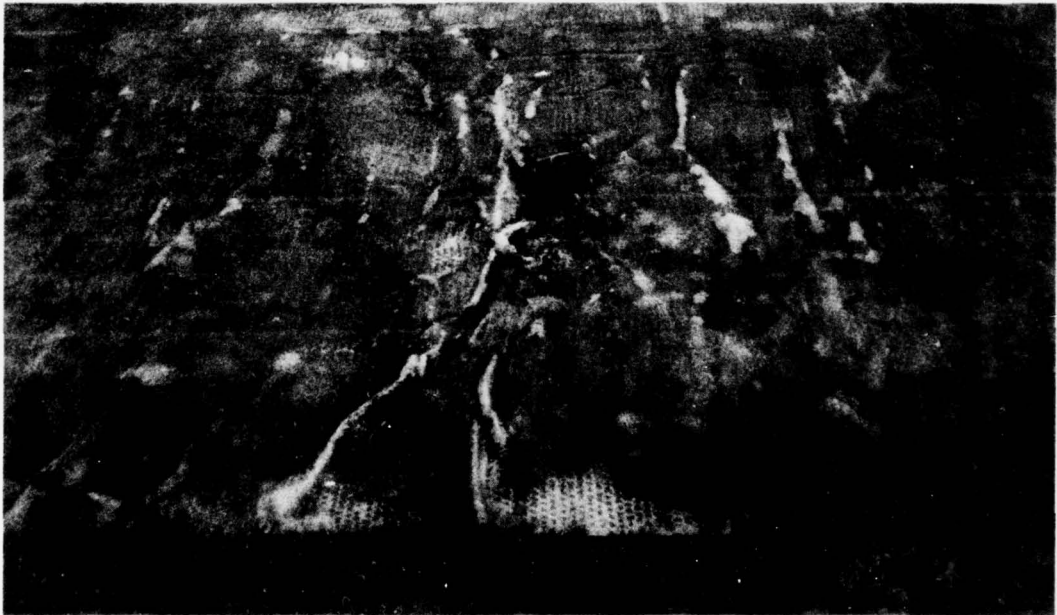
Figure 14. Area with wrinkled fiberglass matting.
