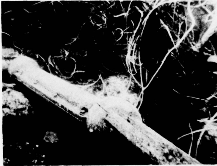
Figure 6a. Damaged pipe showing tangled multiconductive cable.
