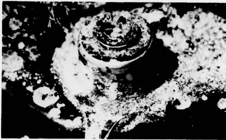
Figure 2a. Cathodically protected fastener from pipe section 57, June 1977.
