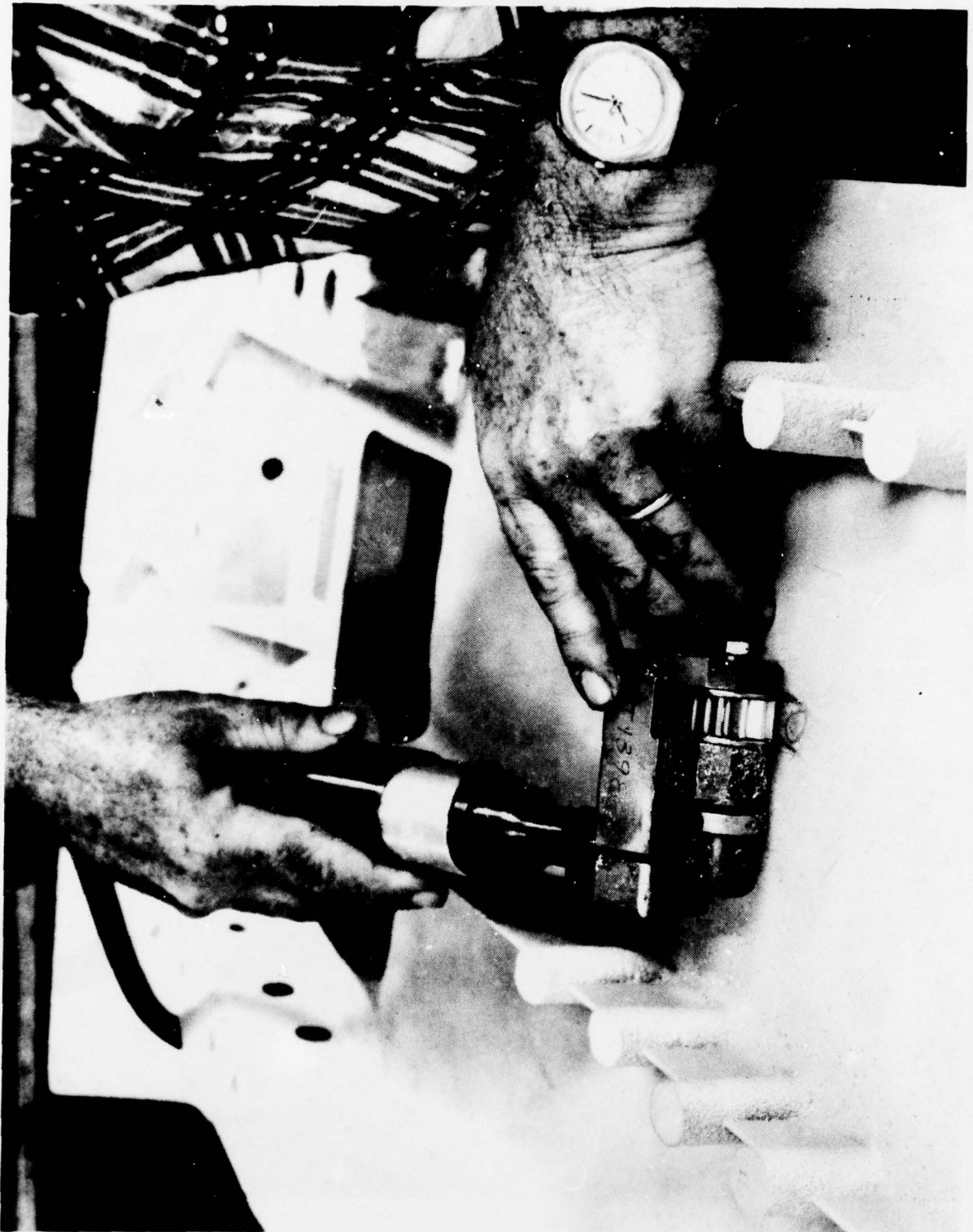
FIGURE 144 BEAD SHAVING EQUIPMENT FOR CLEANING CORRECTED AREA AFTER WELDING
