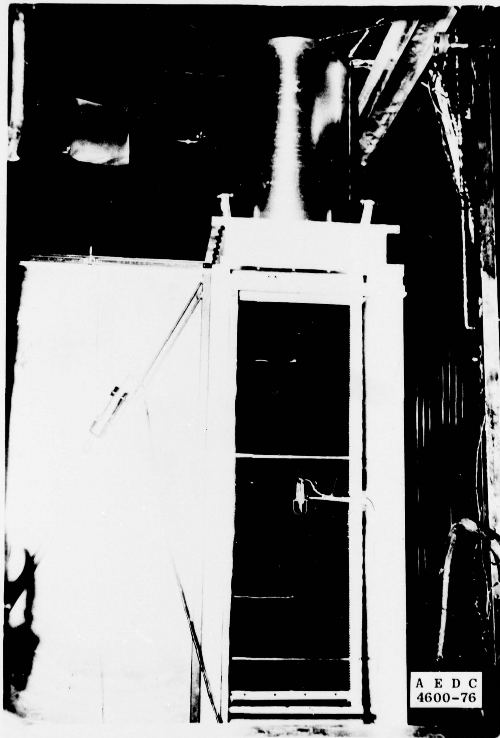
Fig. 6 Type A Cryopump Installation in 12V Chamber.
