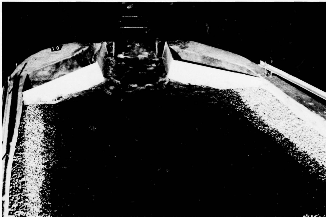
Photo 11. Flow conditions in exit channel, recommended design; pool el 675, tailwater el 582.5, discharge 8,000 cfs
