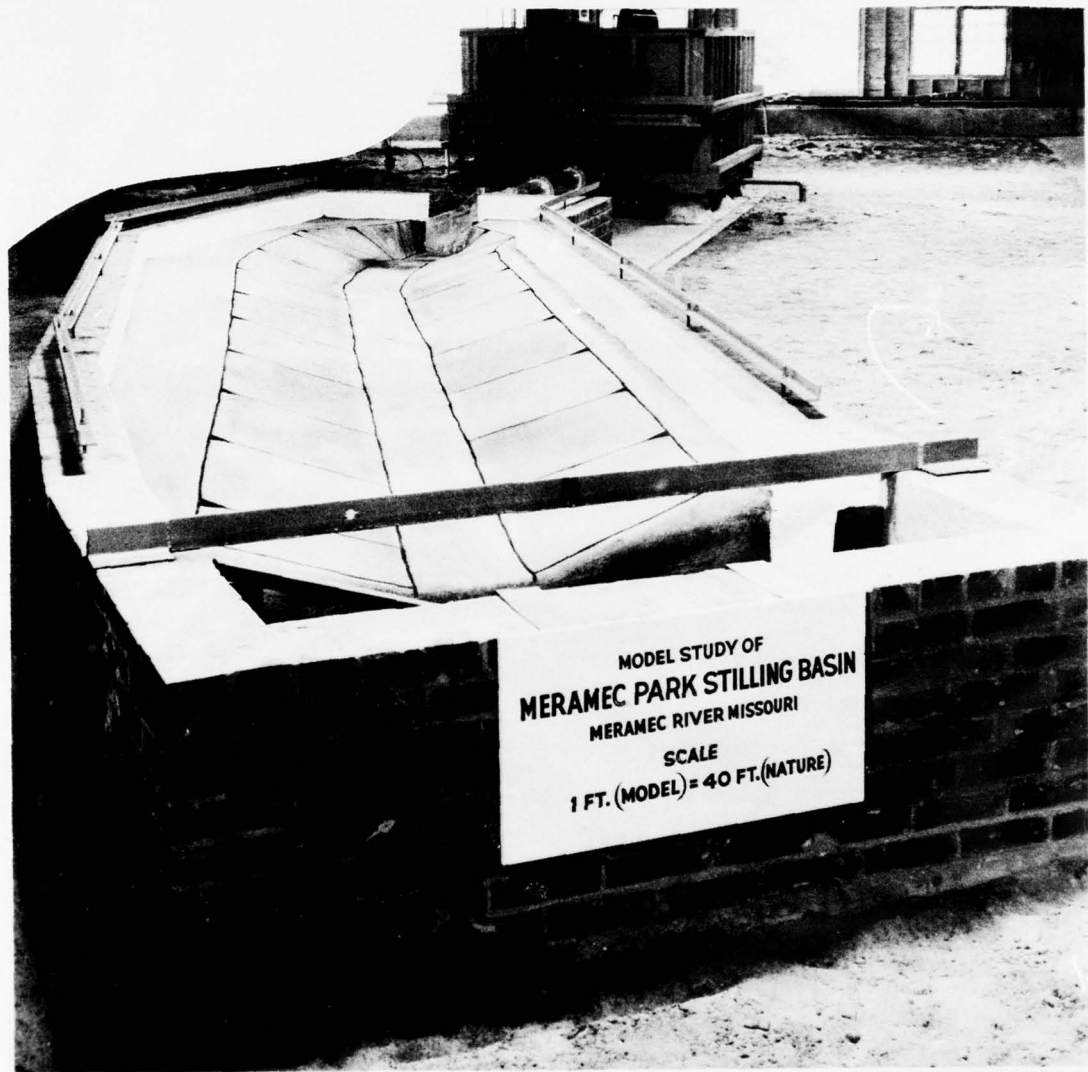
Figure 2. The 1:40-scale model (looking upstream)
