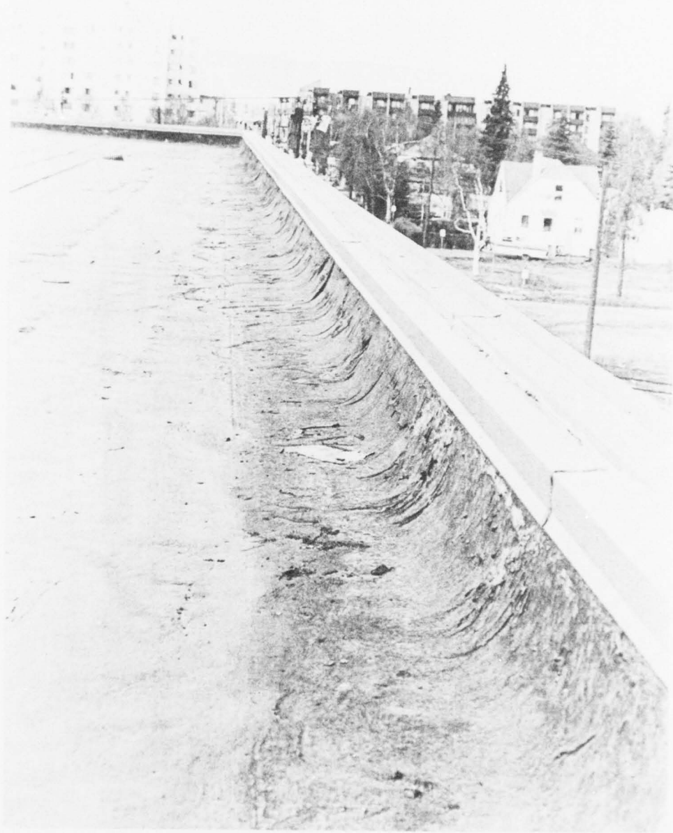
Figure C9. Parapet Wall, Looking North, 11 May 1978.
