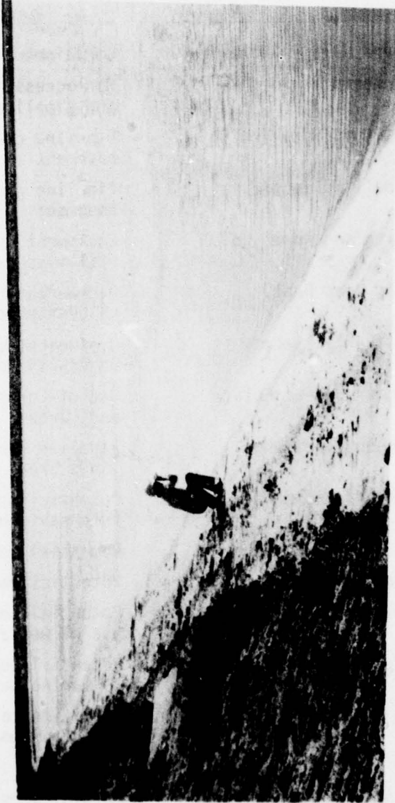
Figure 12. Shrimp culture pond in Containment Area No. 85 showing berm and beach caused by wave action. Such berms protect the levee from further erosion.
