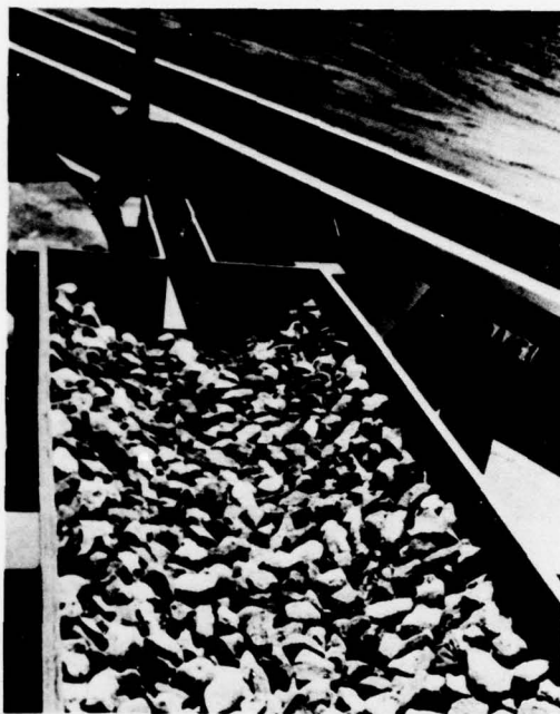
Photo A2. Close-up of diversion channel
