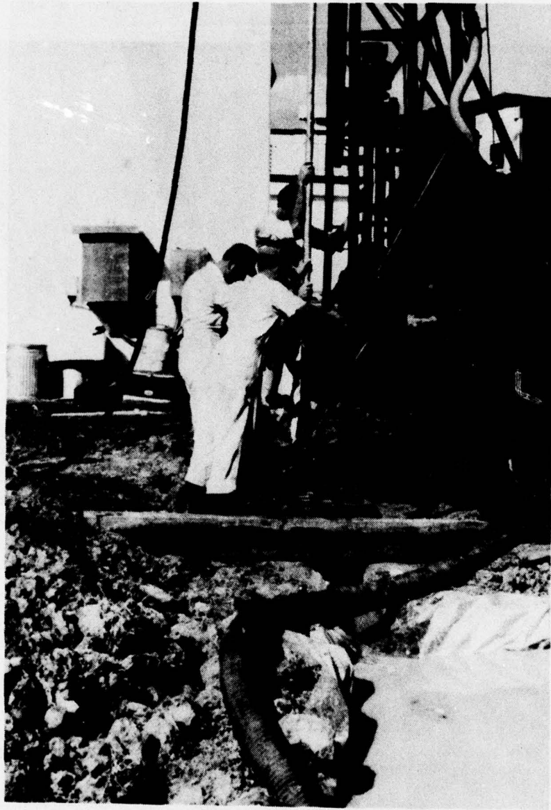
Figure 1. Fluidizing Clay in the Well
