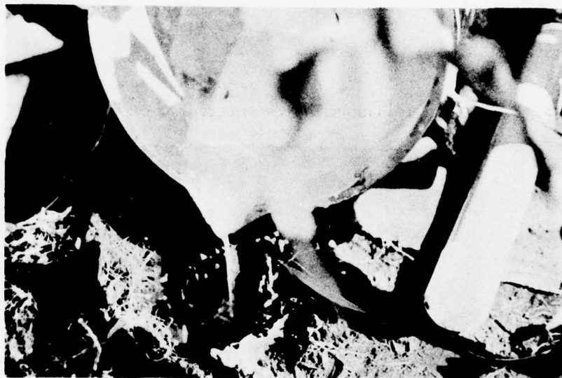
Fig. 10. Pouring a silica flour slurry in the hole.
