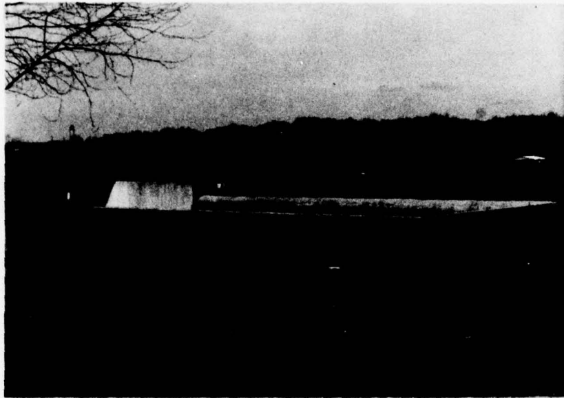
VIEW OF DAM SPILLWAY, LOOKING SOUTHWEST
