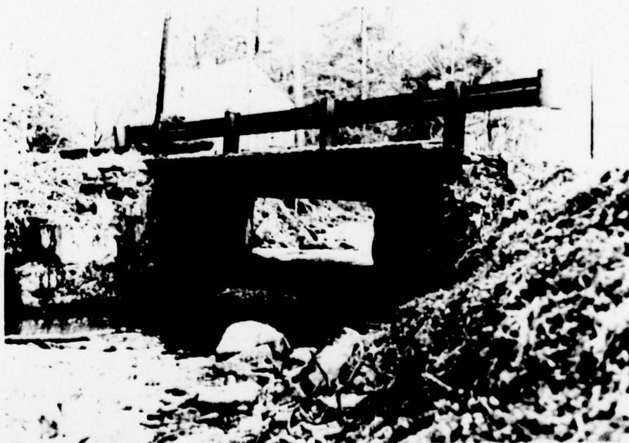
Photograph No. 12 Bridge on Dalton Run Road (Bridge No. 4).
