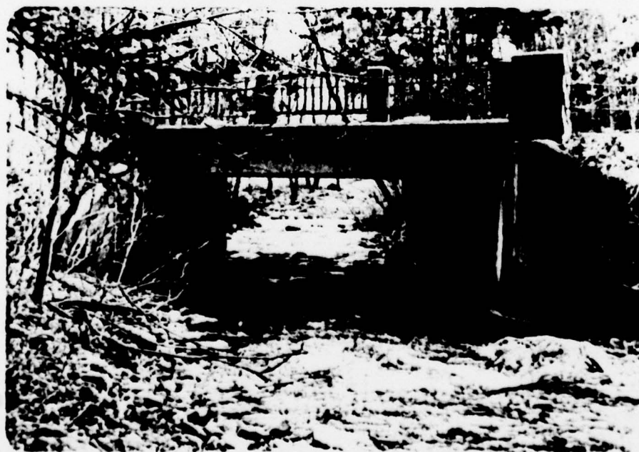
Photograph No. 14 Bridge on County Road (Bridge No. 6).
