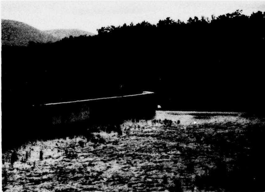
Spillway Below Bridge
