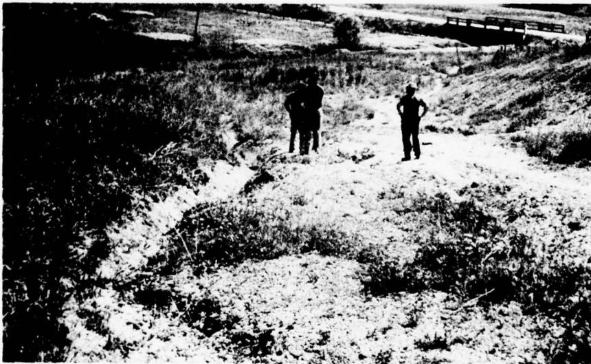
SPELLWAY CHUTE SHOWING EROSION ON LEFT SIDE.
