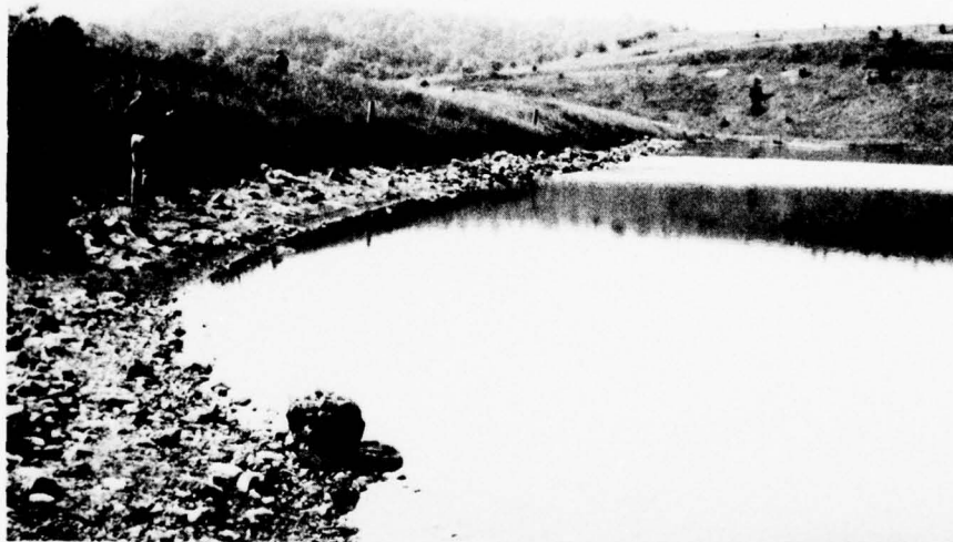
UPSTREAM FACE OF DAM SHOWING RIPRAP FAILURE AND SEVERE EROSION OF THE SLOPE June 1978
