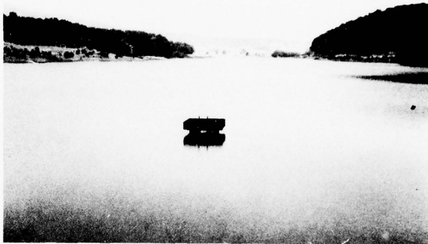
DROP INLET INTAKE STRUCTURE June 1978
