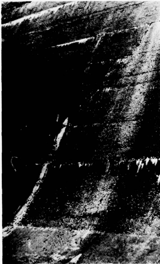
VIEW OF SEVERE DETERIORATION OF CONCRETE ON LEFT ABUTMENT
