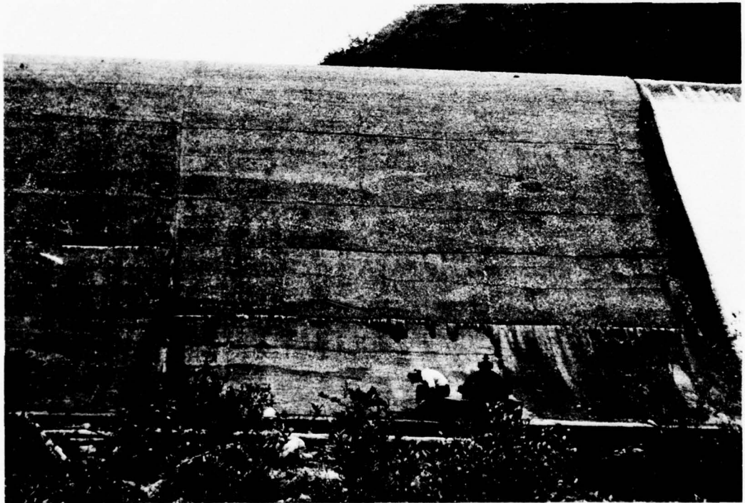
PHOTO 2 Center Downstream Face of Dam
