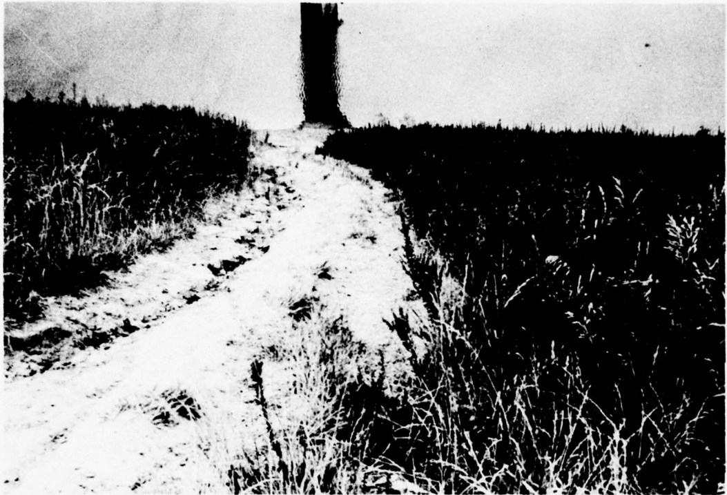
PHOTO 3. Erosion on Footpath - Dam Crest to Water Edge
