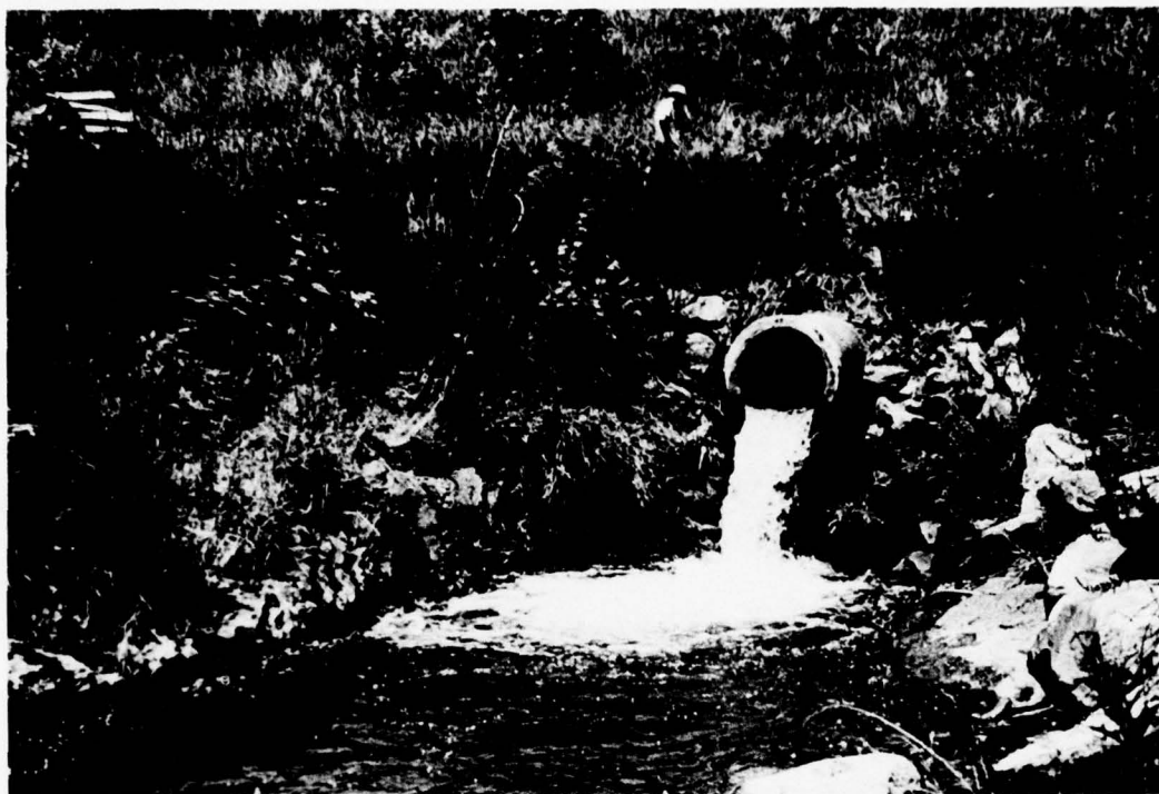
PHOTO 1. Principal Spillway Outlet - Stilling Basin
