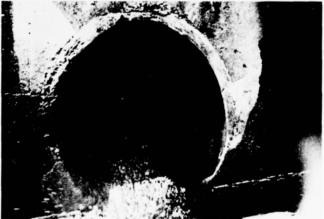
PHOTO 4. View of Outlet of 36 Inch Diameter North Control Conduit
