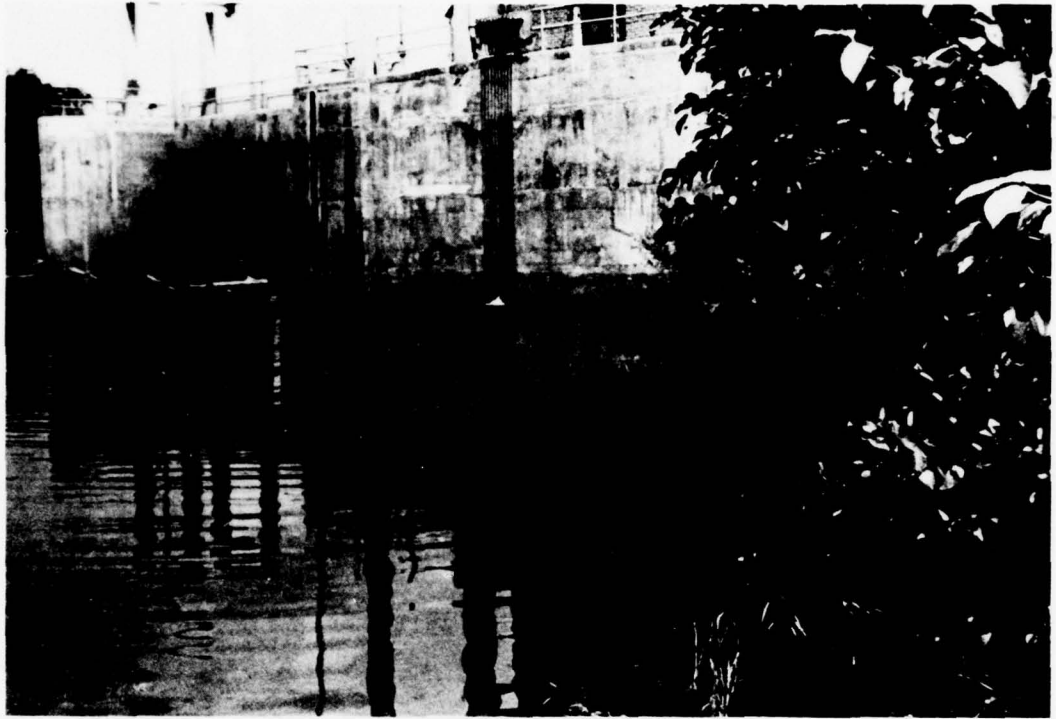
PHOTO 3. View of Upstream Face of Right Non-Overflow Section Directly Above Sluice Gates
