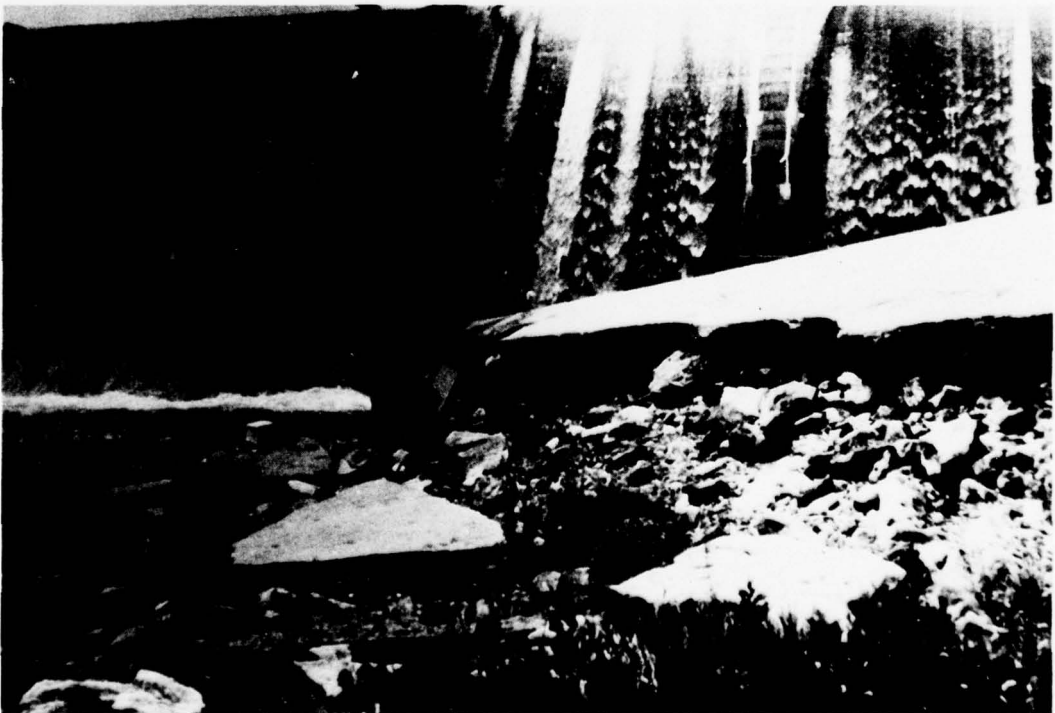
PHOTO 6. View of Deteriorated Concrete Apron Downstream of Left Abutment Area
