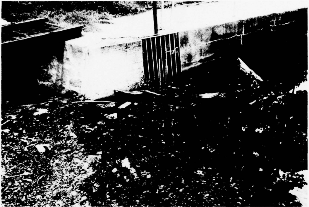
PHOTO 5. View of 30 Inch Intake Pipe and Trash Rack Adjacent to Emergency Spillway
