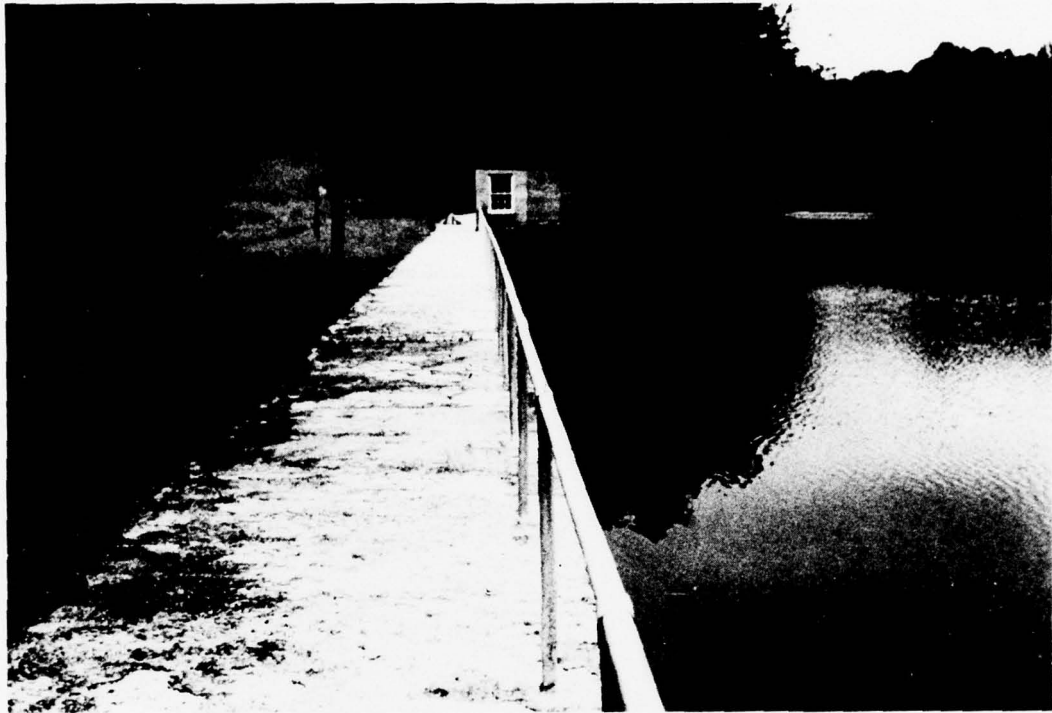
PHOTO 1. View of Dam Crest, Gate House and Reservoir From Left Abutment
