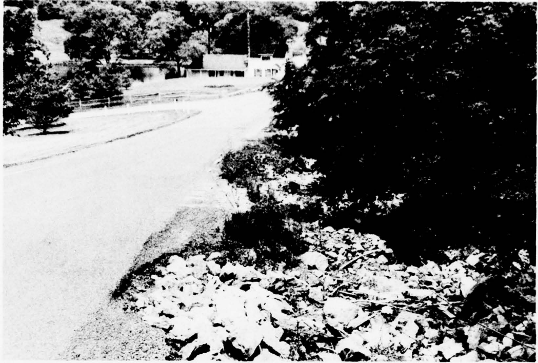
PHOTO 5. Looking Downstream at Emergency Spillway From Point in Line With Centerline Bearing
