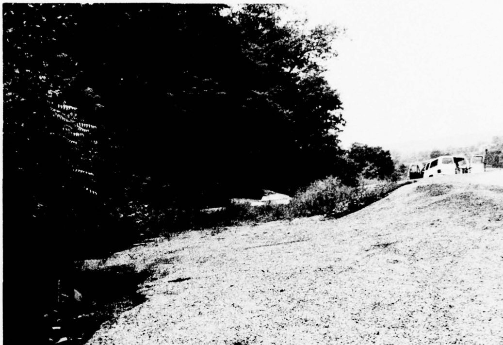
PHOTO 3. Looking Upstream at Emergency Spillway From About 100 Feet Downstream
