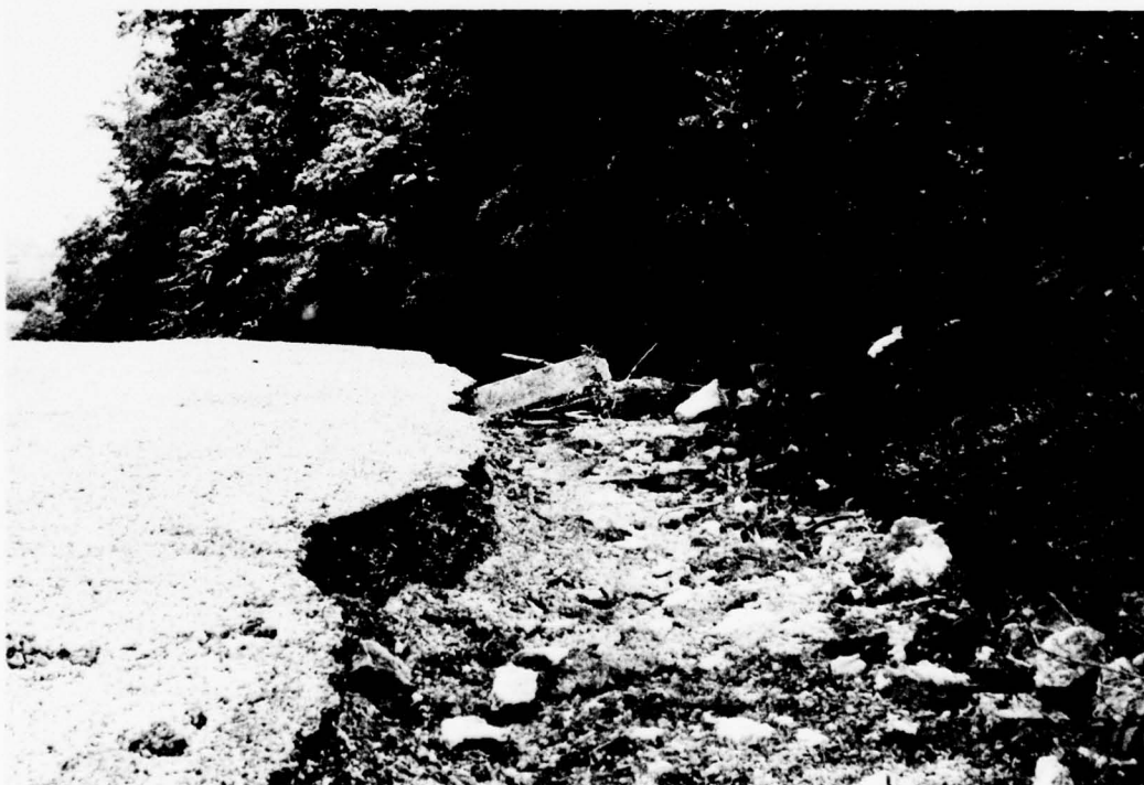
PHOTO 4. Looking Downstream at Emergency Spillway, 100 Feet Downstream From Crest
