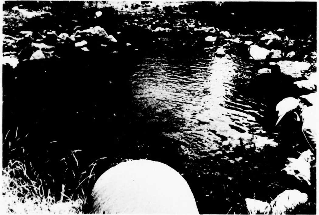
PHOTO 4. Outlet Pipe and Stilling Basin
