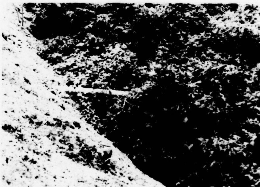
OUTLET PIPE FOR TOE DRAINAGE
