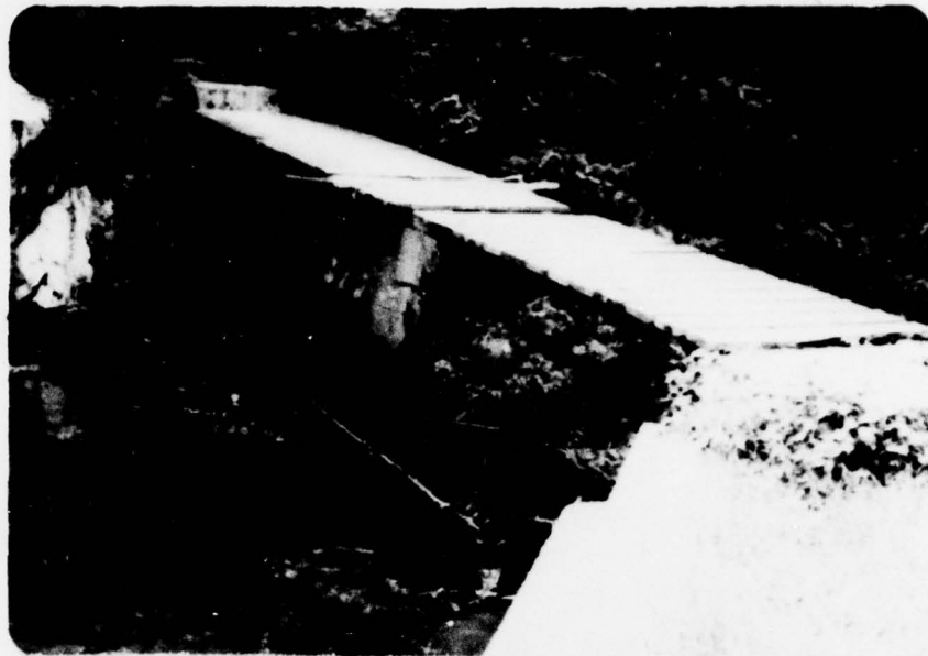
OVERVIEW OF SPILLWAY
