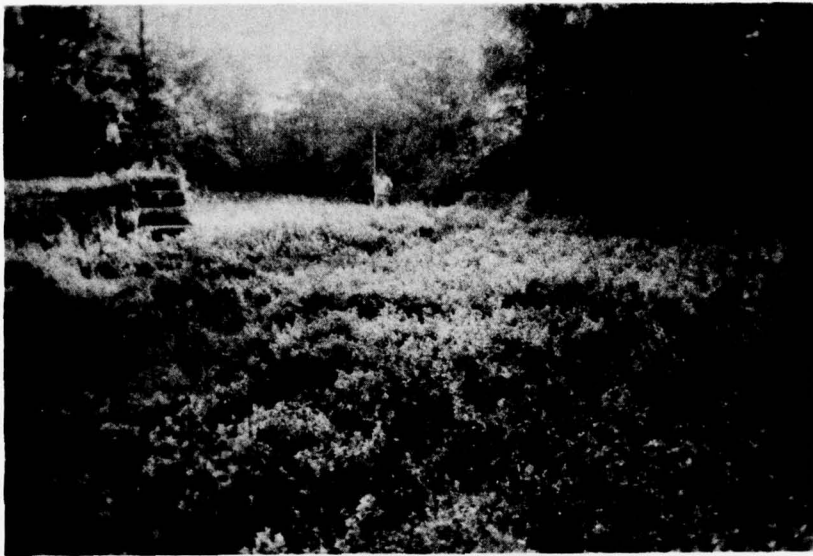
E. Spillway Approach Channel — Looking Downstream.
