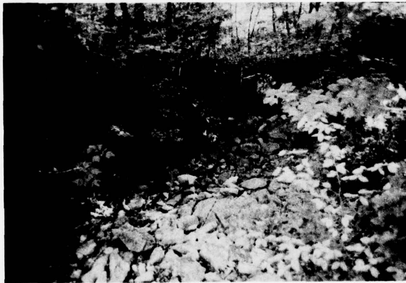
H. Spillway Outlet Channel Below Concrete Weir — Looking Downstream.
