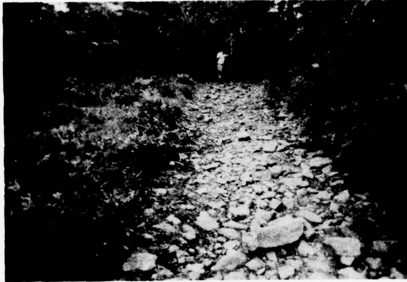
G. Spillway Outlet Channel — Looking Downstream Towards Concrete Weir.
