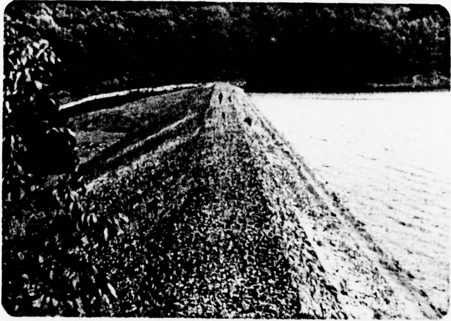
Photograph No. 1 Crest (looking south).
