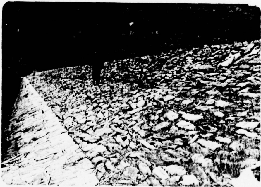
Photograph No. 2 Upstream face.
