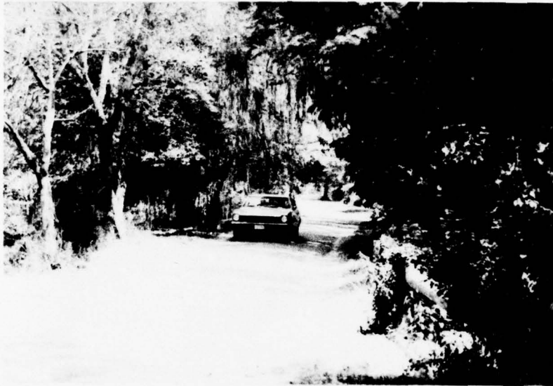
Top of dam east view
