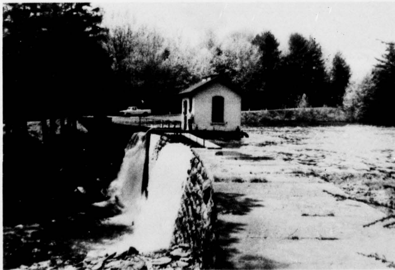
B. Downstream Face of Dam. Looking Toward Right Abutment.
